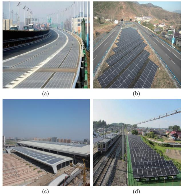
Fig. 5. Scenarios of solar energy-powered transportation. (a) Covered land. (b) Tunnel median. (c) Station rooftop. (d) Trackside land.
